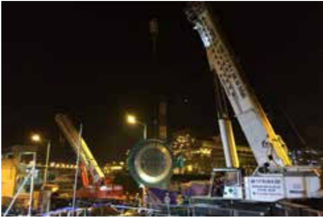
Installation of Tie Valve Mong Duong 2 Thermal Power Plant
