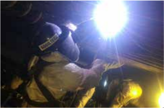
Steam Piping Repair - Mong Duong 2 Thermal Power Plant
