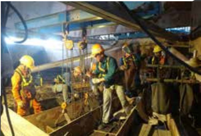
Absorber heat exchangers Replacement Mong Duong 2 Thermal Power Plant
