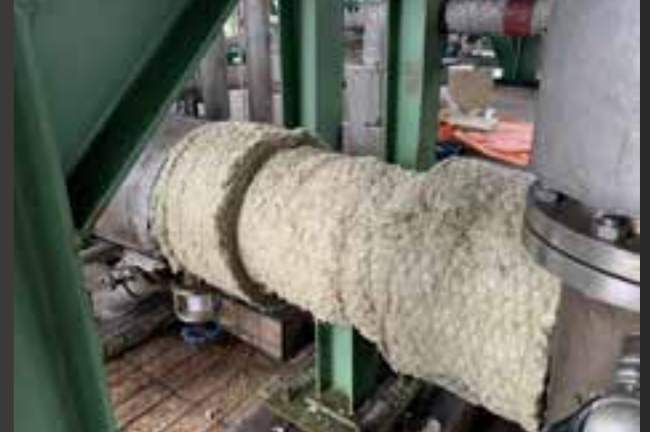
Insulation Installation (TA) Thai Binh 1 Thermal Power Plant
