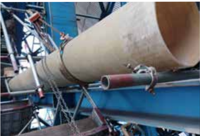
Fabrication & Installation Ash Chute U1, 2 Mong Duong 2 Thermal Power Plant
