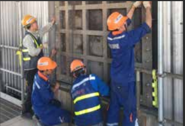
Absorber heat exchangers Replacement Mong Duong 2 Thermal Power Plant
