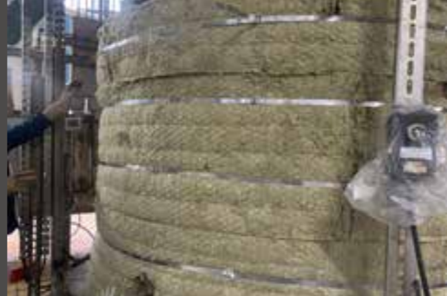
Insulation Installation (TA) Thai Binh 1 Thermal Power Plant
