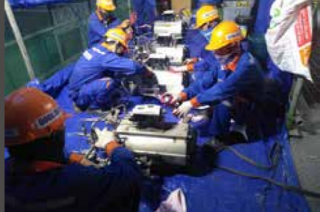
Maintenance for Control valve & Actuator Mong Duong 2 Thermal Power Plant
