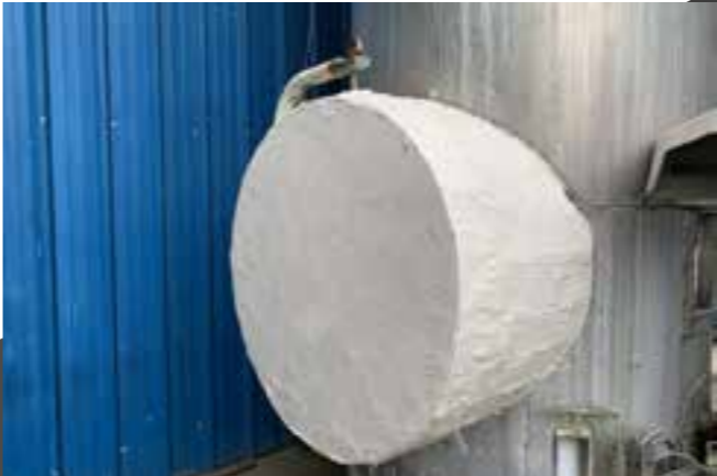
Insulation Installation (TA) Thai Binh 1 Thermal Power Plant
