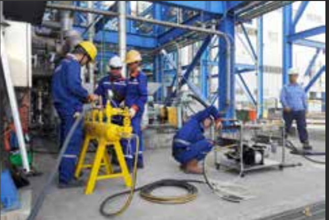
Hydro test AUX. Boiler & Deaerator Tank Mong Duong 2 Thermal Power Plant
