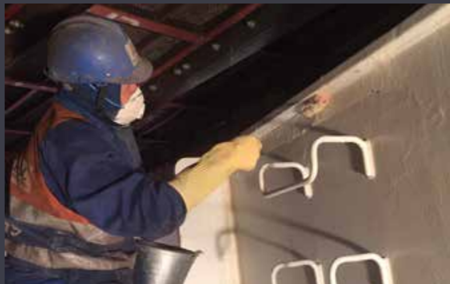
FGD, SCR, Absorber (Flake Lining) Blasting and painting Ceilcote Ha Tinh Formosa Project
