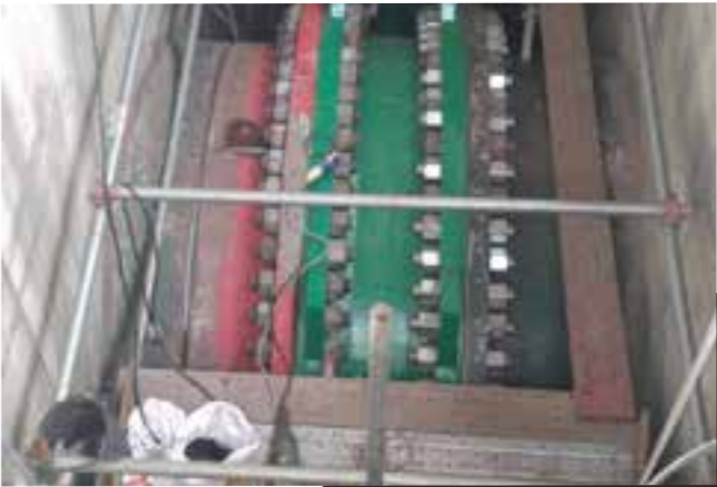
Installation of Tie Valve Mong Duong 2 Thermal Power Plant
