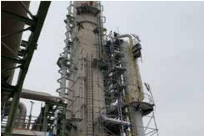
Scaffolding Erection Thai Binh 1 Thermal Power Plant
